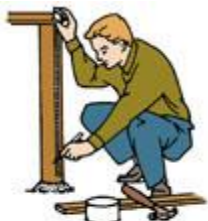
Measure from the top rail to align each bottom rail on each post.
