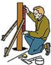
Use a level to make sure each post is in an exact, upright position.
