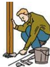
Build a mound around each post to eliminate standing water.
